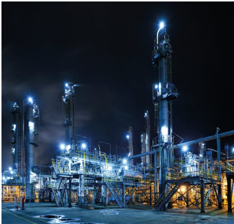
Illustration 1: Cutting-edge LED technology for the illumination of industrial installations has to be efficient as well as temperature-resistant
