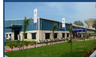
Production Site, Chennai
