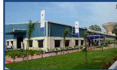
Production Site, Chennai
